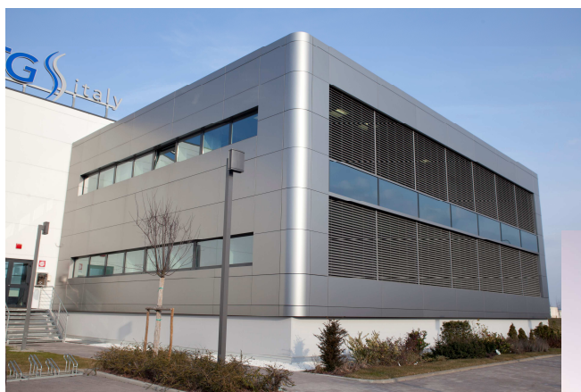
Parete ventilata coibentata in Alucobond
