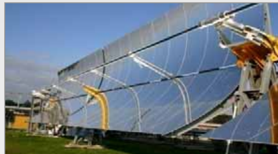
Test facility PCS
